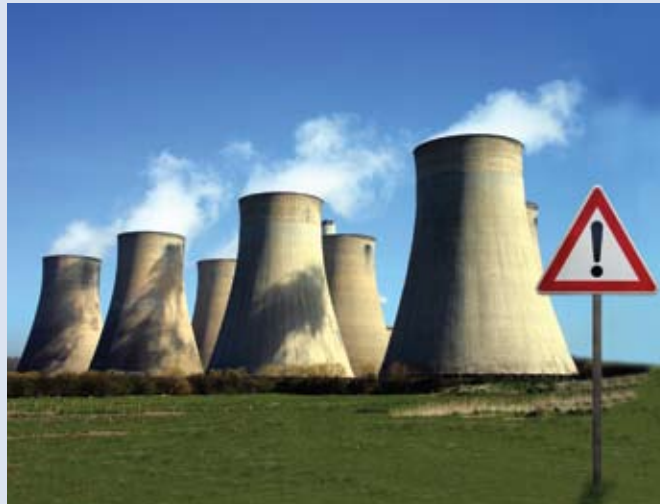
Cooling Towers of coal fired power station
